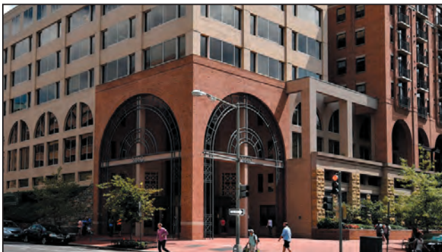
Façade of 2440 M Street façade before demolition.
